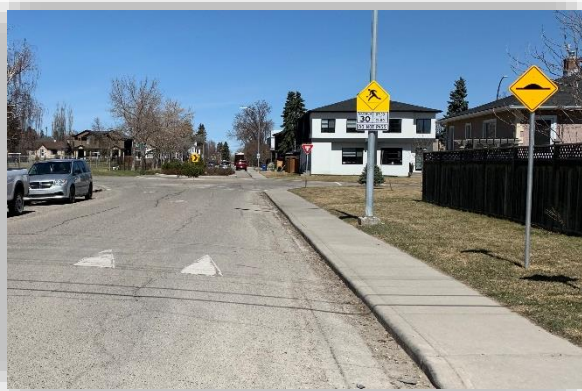
Additional speed humps
