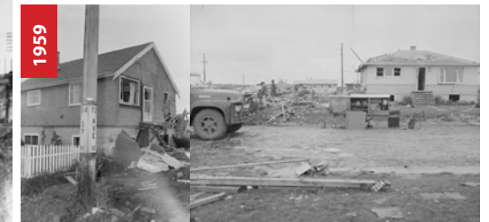
Aftermath of house explosion in 24 Street and 72 Avenue SE [left CU1132021 & right CU1131907].
