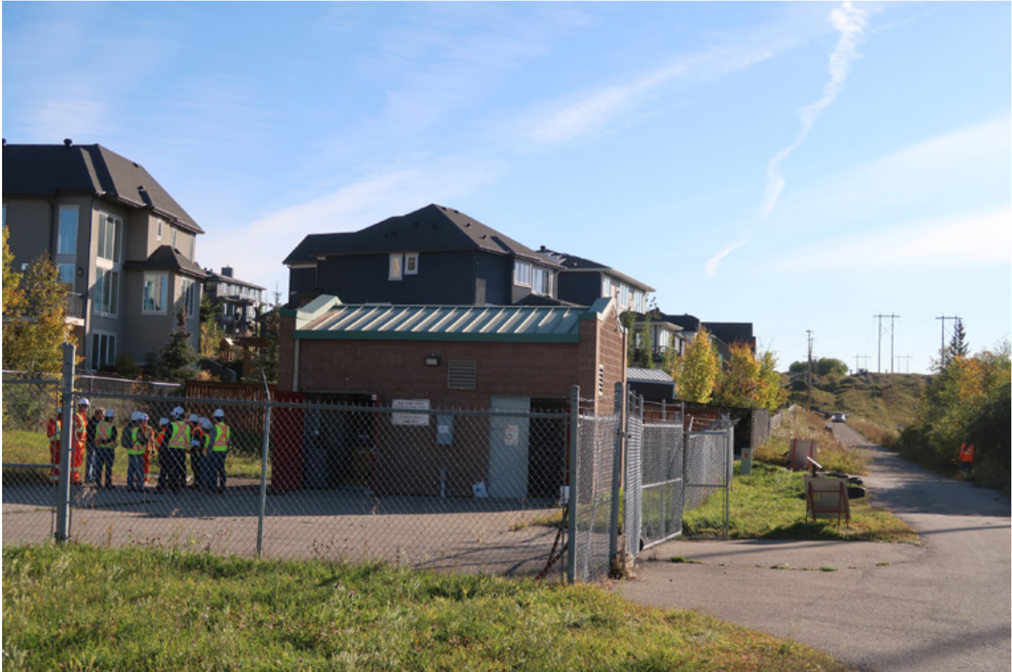
Existing Lift Station
